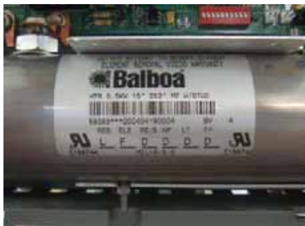
Heater Element Specifications Are Shown on the Heater Tube Label
