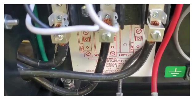
As we are using 240V you also need to move two cables over. The Blue Cable (which is the pump) and the Red & White Stripe Cable (which is the blower) need to move from the neutral connector, over to the Line 2 as shown in the photograph below. (Solid White cable stays where it is)
